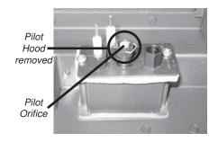
Remove the pilot orifice with the allen key.
